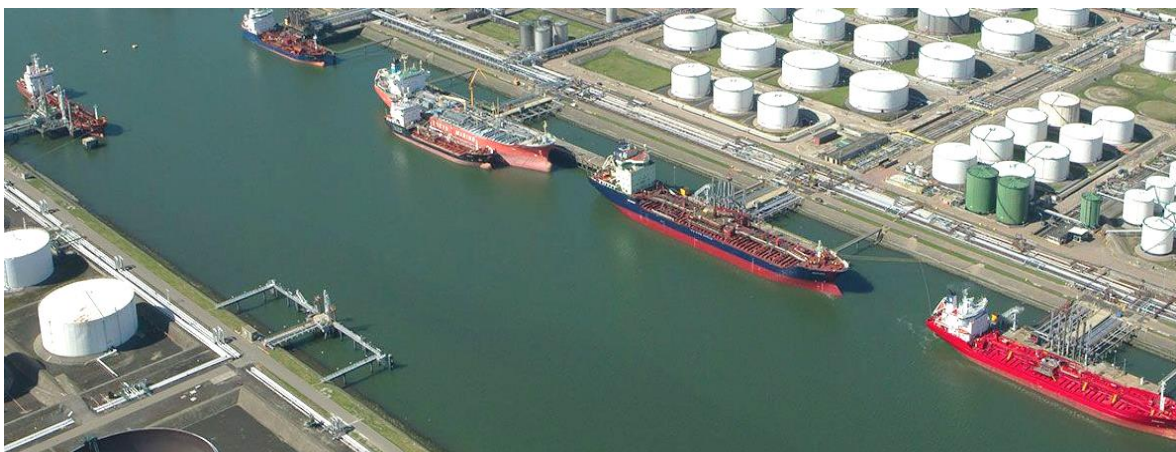
Typical mooring at sheltered berth
